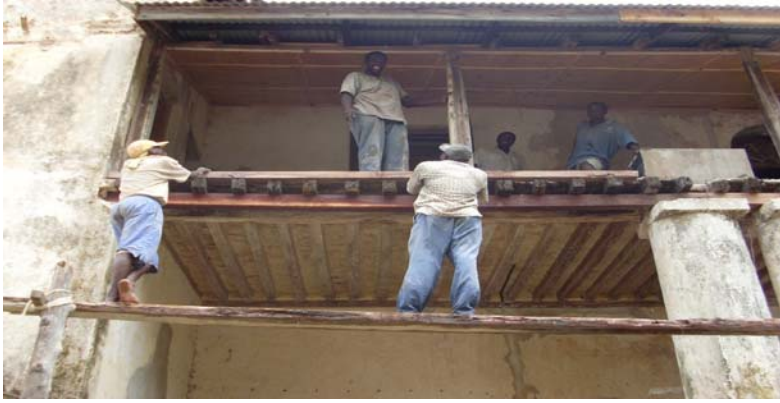
REPLACEMENTS OF MAIN BEAM
