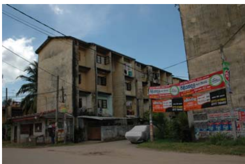
Common rear space has been used to construct another house
