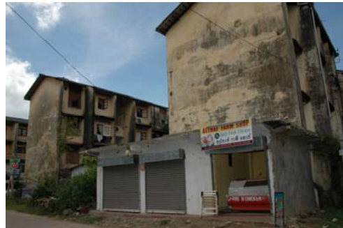
Ground floor house has been extended & constructed three shops.
