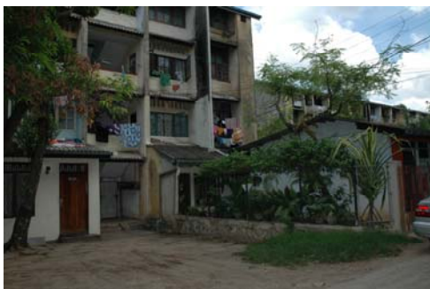
No proper lighting & ventilation due to unauthorized constructions
