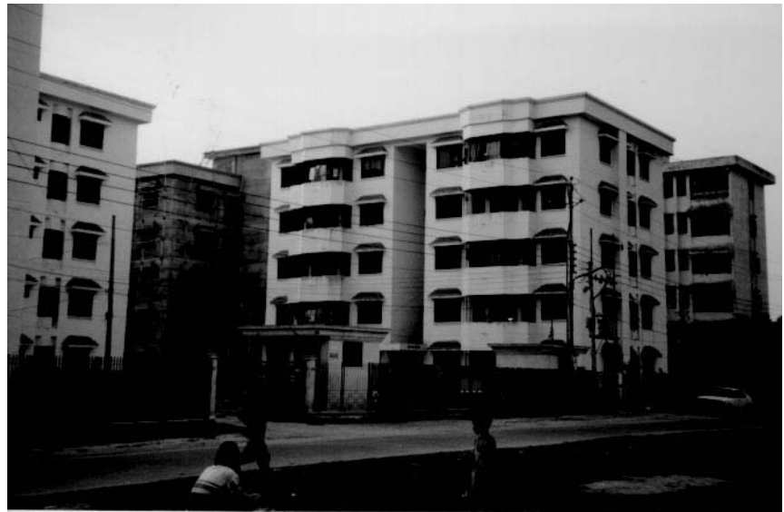
Photo 2: "E" Type New Building in Region G at Azimpur Governmental Housing Area
