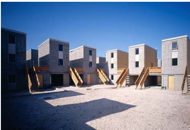
Fig. 7 : View on original buildings( Elemantal, 2005)
