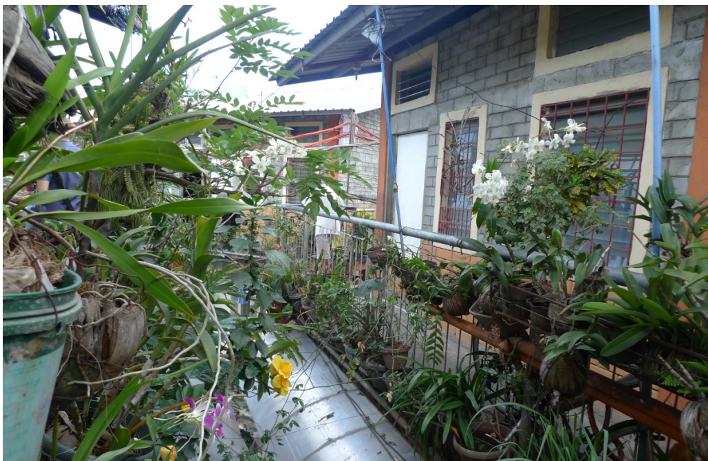
3. The hanging gardens of the access balconies
