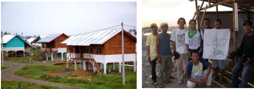
The housing typology is a detached house on stilts. The villagers present the result of community mapping. Pictures http://www.architectureindevelopment.org/project.php?id=297
