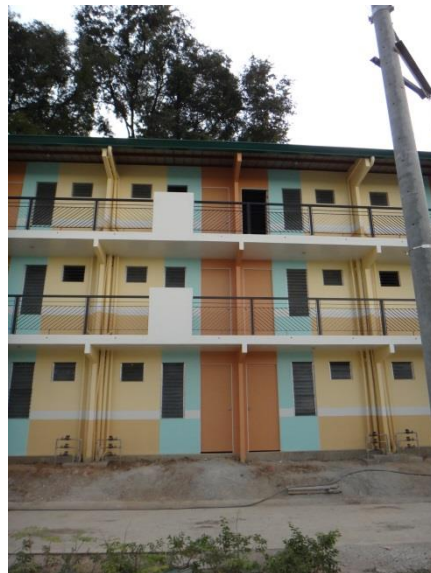
Photo 5: Plaster and painted concrete shell structure at Bistekville 2
