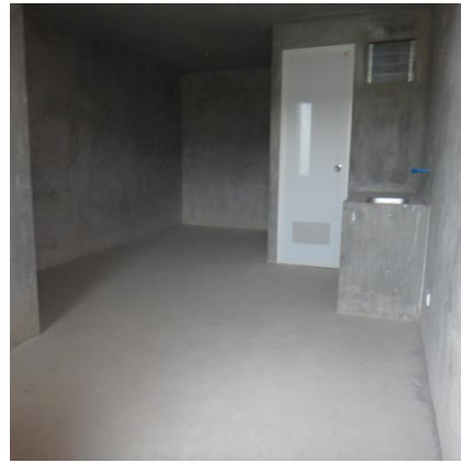
Photos 8 & 9: Housing units in Bistekville 2 - exposed concrete finish, lack of natural ventilation
