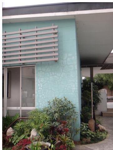
Photos 6 & 7: Deteriorating concrete at Sofia Bellevue & Smokey Mountain
