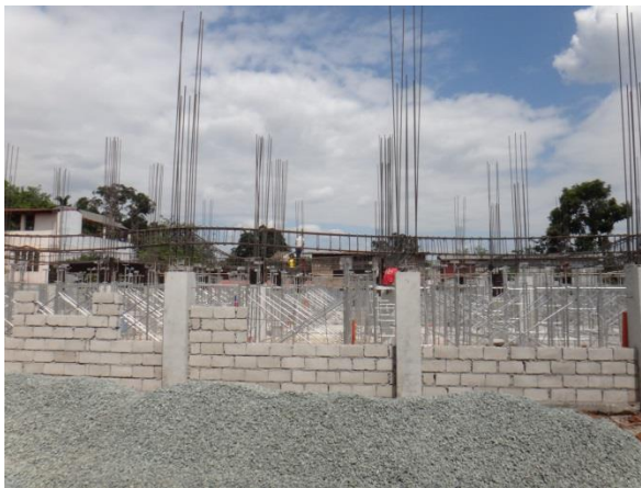
Photos 3 & 4: Reinforced concrete with CHB construction & cast insitu shell concrete construction
