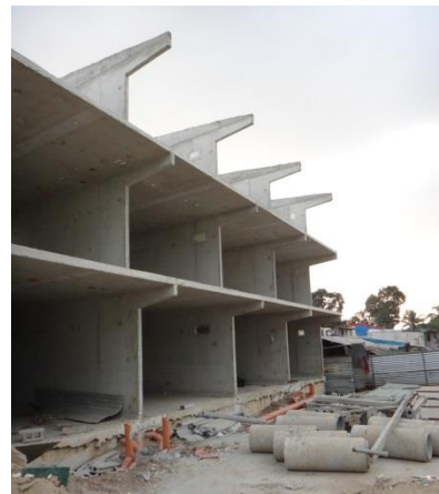
Photos 3 & 4: Reinforced concrete with CHB construction & cast insitu shell concrete construction
