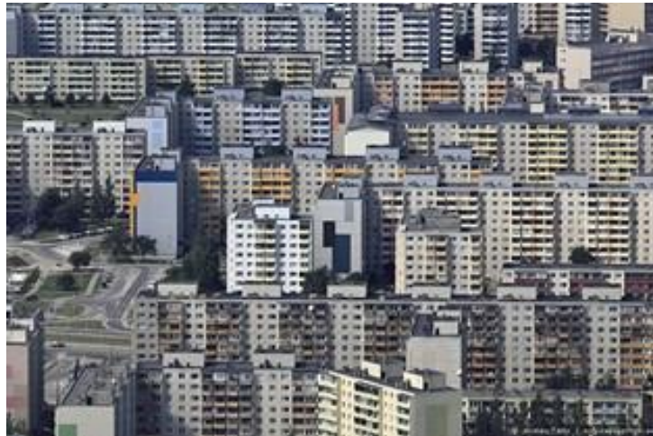
Photo 1: Rise of concrete towers, http://www.efla2011.com/program/technical-tours.html
