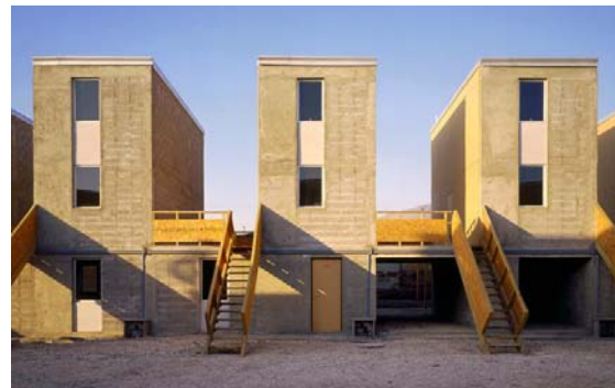
Figure 4. Quinta Monroy as initially provided. (Elemental)
