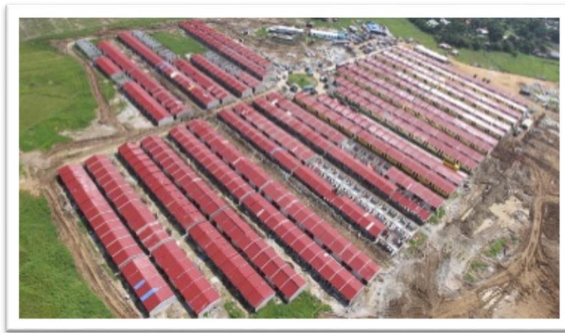
Monofunctional rowhouse relocation project
