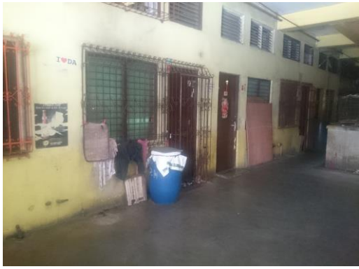
Illustration 8. Smokey Mountain, Metro Manila. Project by: NHA. Sense of control/security achieved by the use of metal fences in windows and doors. (photo: DARC)
