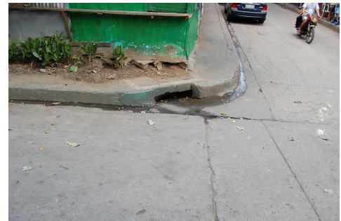
Underground stormwater channels without grills (photo taken by the author)
