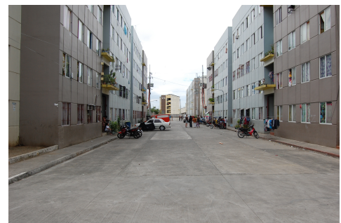
Impervious paving causes instant and fast run-off flows (photo taken by the author)
