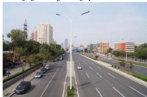
Wide road for cars and there is no lanes for bikes Photograph: Personal
