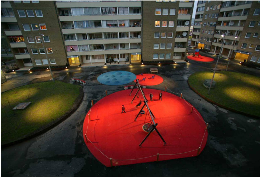
One of the upgraded courtyards (One size doesn't fit all, 2009)
