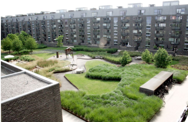
Figure 5. Large semi-enclosed courtyard in Charlottehaven, Copenhagen by SLA (Landzine)
