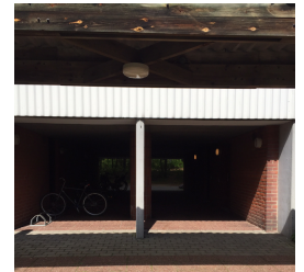
Picture 3: Openings between the courtyard and cycle path. This make a connection between these to rooms.
