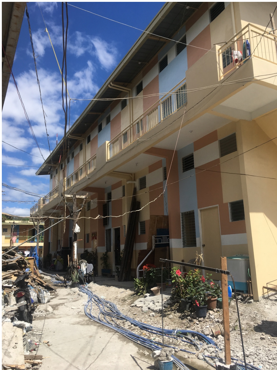
Bistekville 4 under construction. (Photo: Wiberg)
