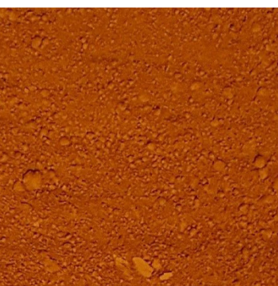
Pigmented concrete Floors on exterior corridors.
