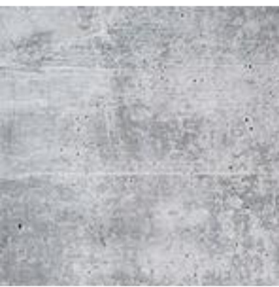
Raw concrete Framework, walls and floor.
