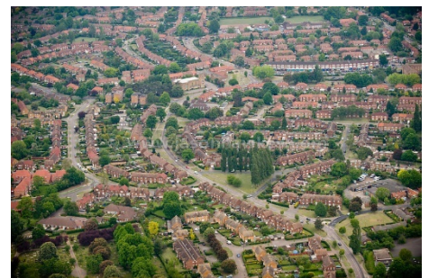
Picture 2. Welwyn Garden City, that was completely designed after Howards principles and the Garden City movement.
