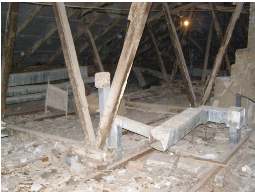
Venilyation system destroyed, chemneys are removed, the rested are deteriorated
