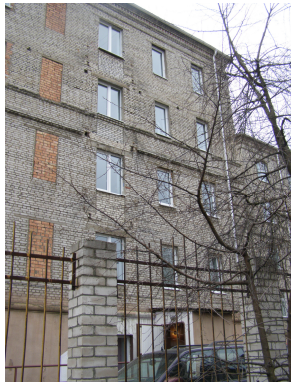
Leakadge on the outer walls, the plot is not paved well, the fence is unfinished
