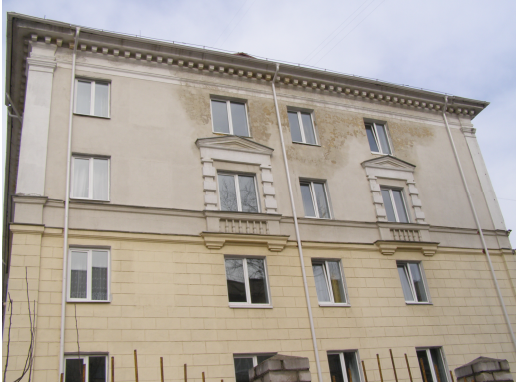
Leakadge on the outer walls, the plot is not paved well, the fence is unfinished
