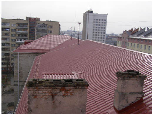
Venilyation system destroyed, chemneys are removed, the rested are deteriorated
