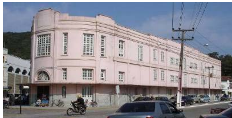
Figure 10: West façade view (2007)
