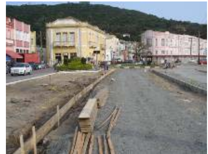
Figure 19: Pavement renewal with concrete blocks (september, 2007)
