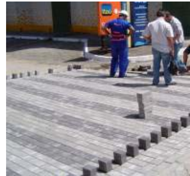
Figure 18: Pedestrian stripes being executed (2007)
