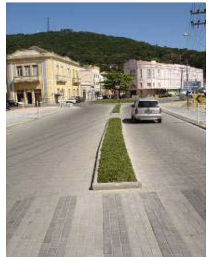
Figure 20: Finished new pavement with concrete blocks (january, 2008)
