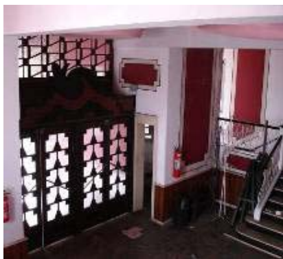
Figure 14: Main entrance – Lobby (2007)
