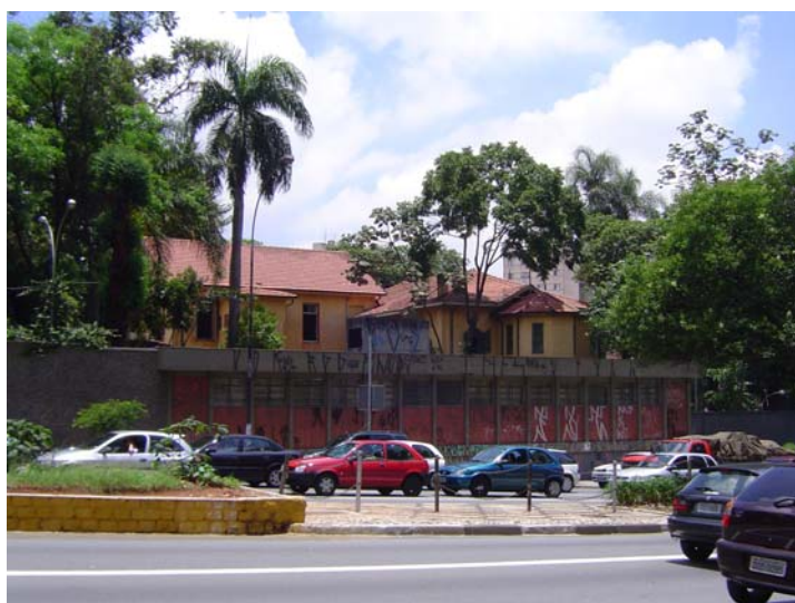
Figure 7: The Lane House completely hidden by the supplementary building built in the 1970s. The demolition of the supplementary building will allow the house to be seen from the street. Photo: Tatiana Cipoli
