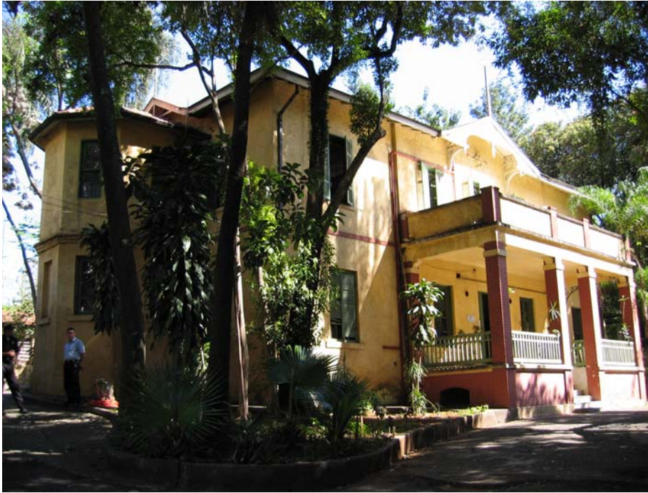
Figure 3: Lane House, main façade (North). Photo: DPH
