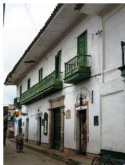
Fig 6 View from calle Ricaurte, Main access.
