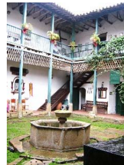
Fig 8 View of the central courtyard.
