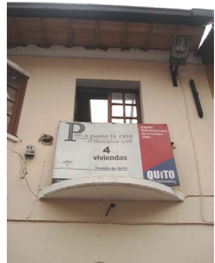
Figures 26: Program tag. 4 apartments are distributed from an single family original house.
