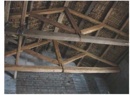
Figures 19: Wood trusses, roof battens and “chacla” system as support of clay tiles covering.
