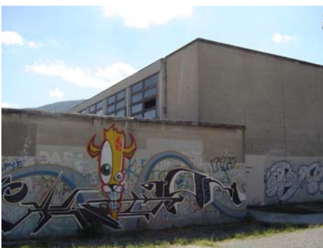
Figure 18. Concrete wall covered with graffiti
