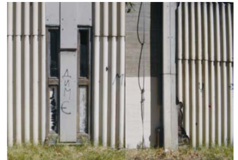
Figure 19. Asbestos cement façade on the gym hall
