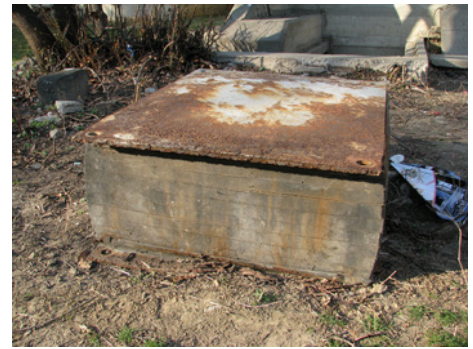
Figure 22. Pneumatic foundation, condition September 2007 and February 2008
