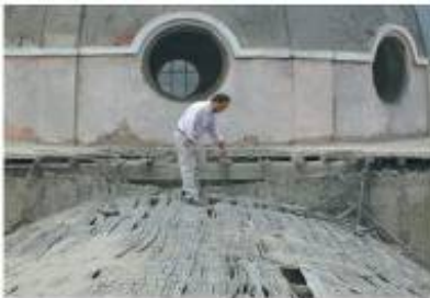
Figure 14. Roof (external part of the vault and dome) in 2003
