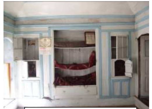
Figure 15: Timber closets in M4
