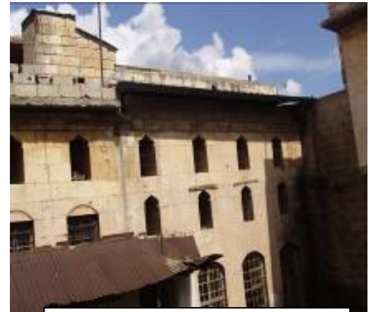
Figure 20: General view of the building
