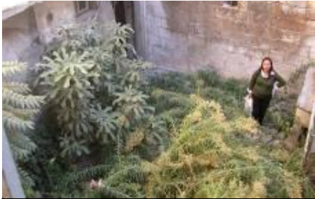
Figure 12: Courtyard before cleaning of vegetation
