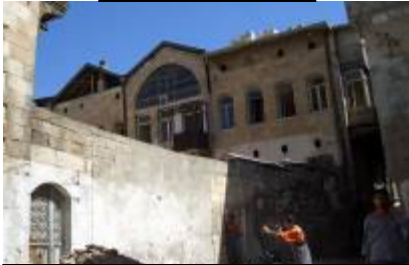
Figure 6: Traditional house from street
