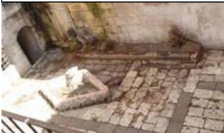
Figure 13: Courtyard floor with Pool after cleaning of vegetation
