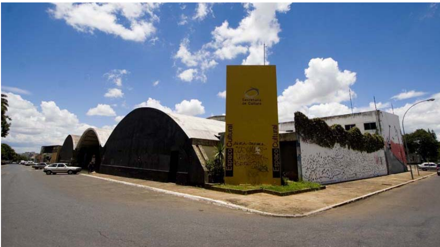
Figura 5: Facade W-2 and lateral facade
