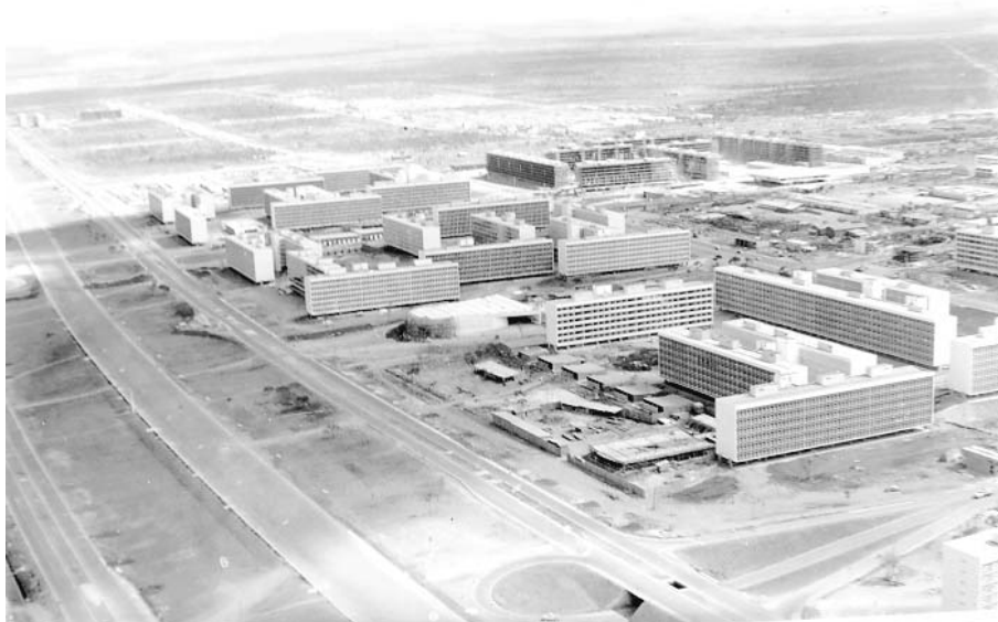
Figure 4: Construction of Superblocks.
