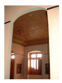
The construction technic used in the building is self sustaining structural wall system with thick walls of red brick. Most of the roof is a wooden structure covered ceramic tiles, part of it is accessible and now used as a terrace, patio floors are of stone and rooms floors are of wood.
