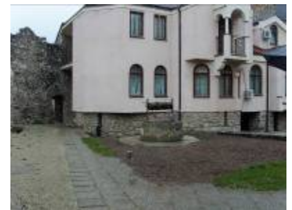
Figure 38: Present situation in the small court, west side with New hose and small economical gate
