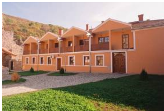
Figure 21: View of the Dionisije's building, small court north wing (2008)
