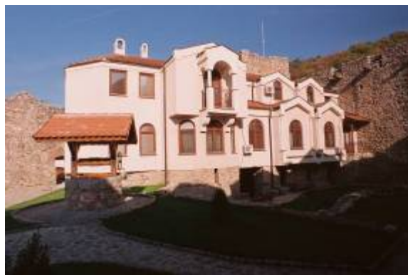
Figure 20: View of the New house built in 1988 above the conserved remains of the workshops, small court north wing (2008)
