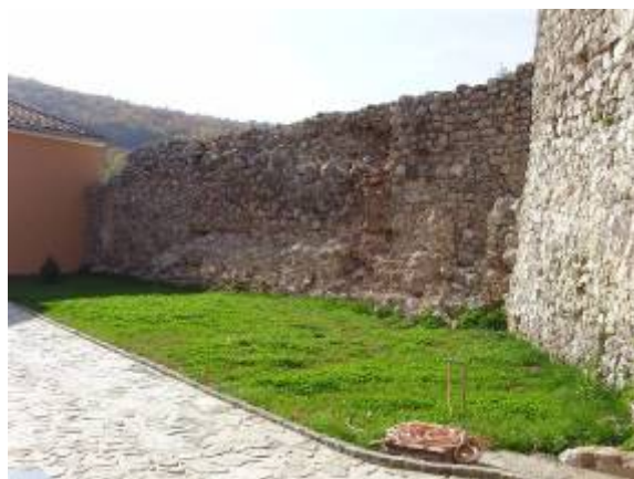
Figure 23: View of the empty space between New house and Dionisije's building (there was one floor guest house, but it was crushed), small court west wing (2008)
