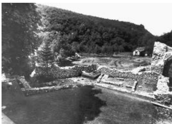
Figure 14: View of the excavated utility objects, main court west wing (1975)
