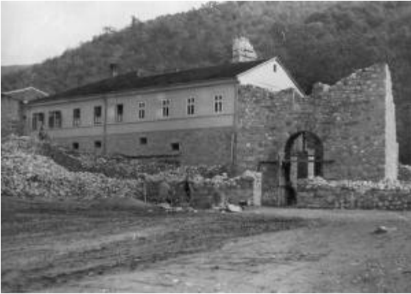
Figure 11: View of the Dionisije's building (1985)
