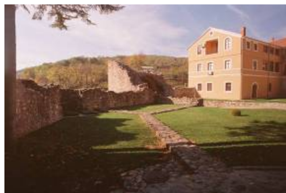
Figure 15: View of the gate tower and remains of medieval objects, main court west wing (2008)
