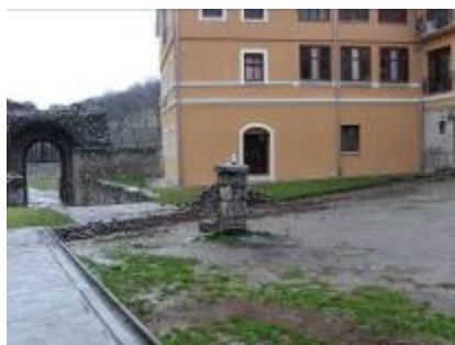
Figure 34: Present situation in the main court, north-west corner
