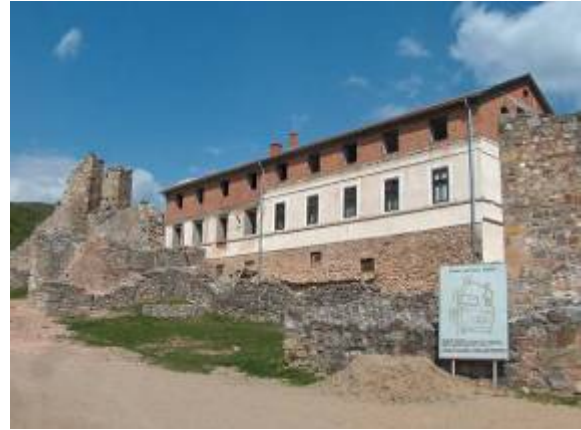
Figure 12: During the building of new second floor (2006)
