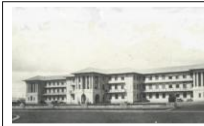
Plate 6: Railway headquarters as completed in 1927. Source: Kenya Railways 1977
