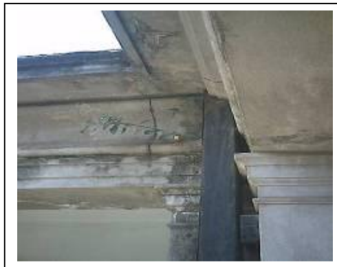
Plate 18: Attack on concrete block and moulding by algae and plants
