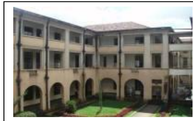
Plate 7; Railway Headquarters internal courtyards Source: Author. 2009
