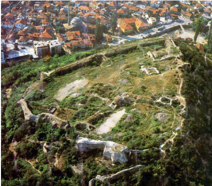
Figure 4: Fortress of Prizren before and after
