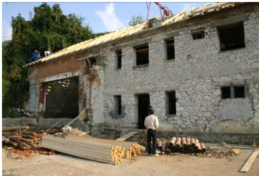
Figure 16: Syndicate building during restoration project in 2006
