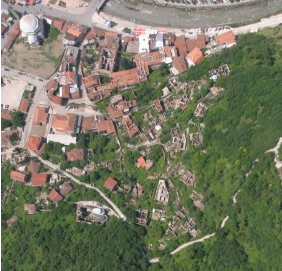
Figure 8: Nënkalaja aerial view after the March riot and destructions
