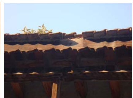
Damage of roof tiles
