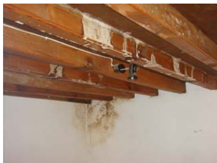
Water leakage from the roof
