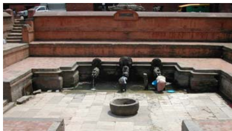
A Traditional Stone Spout dating back to 6 th Century which was repaired and maintained by the Sub-Metropolitan City Office
