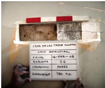
Structural coves – mud and clay
