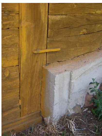
Figure 24. The church, detail of foundation wall
