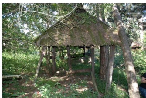
Figure 23. Sobrasice, half-opened type, almost collapsed
