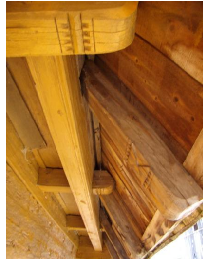
Figure 19. The church, detail of decoration
