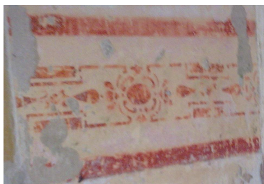
Figure 2: Decorative paints on corridor walls
