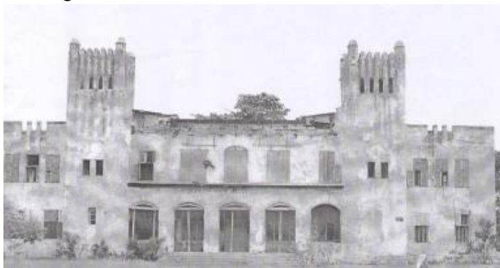
Figure 6: The Front Facade
