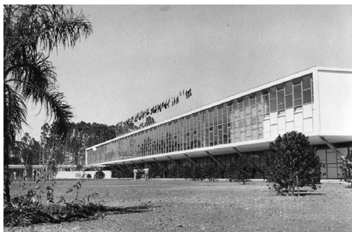
Figure 11: view of Nations Pavilion, when the park was already accomplished.
