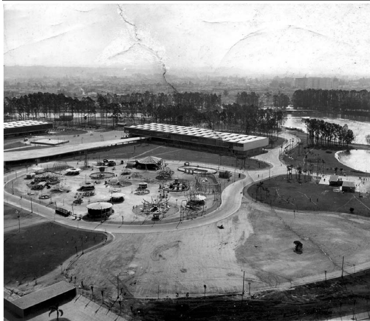
Figure 10: view of the Ibirapuera park, in construction. The Nations Pavilion (today's Afro Museum), is in the center of the picture and the States Pavilion is in the left. Notice that the open area was used by a children leisure park, before its transformation in a green area.
