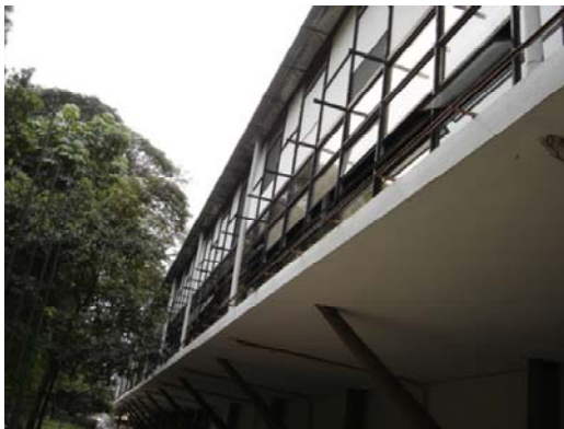
Figures 1 and 2: The ground floor and the first floor in 2006. The original Niemeyer 1953 plan had free floors, with all bathrooms, support and technical functions located in the extremity of the long plan. All internal rooms and the annex, located in the north extremity (left side in this picture) are not original.
