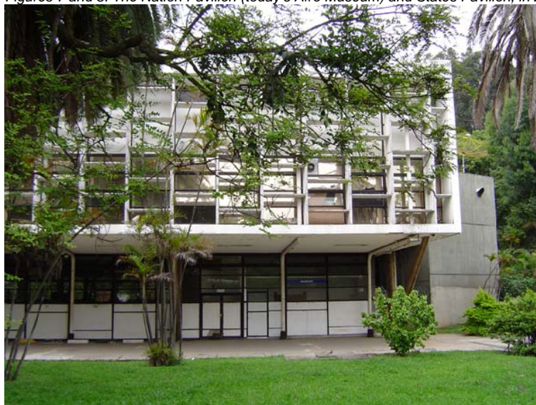
Figure 9: view of States Pavilion, from the main façade, the one that connects to the slab roofing, and that is protected by concrete brise-soleil.
