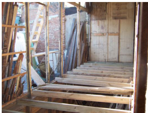
Figure 50. View of structural repair in interior.
