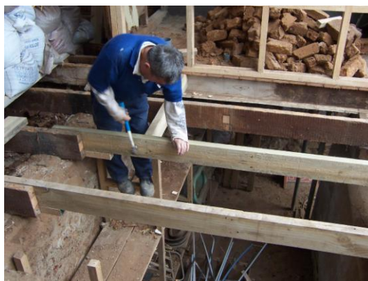
Figure 51. View of structural repair at basement.
