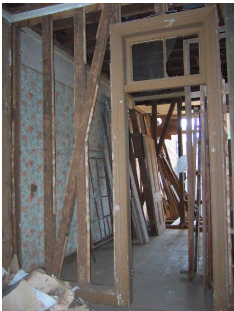
Figure 33. View of interior intervention.
