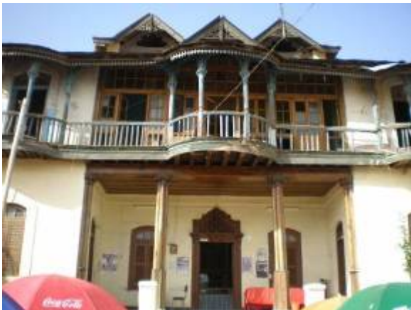
Fig.3.1. The Exterior Wooden Features of the Teferi ouse House
