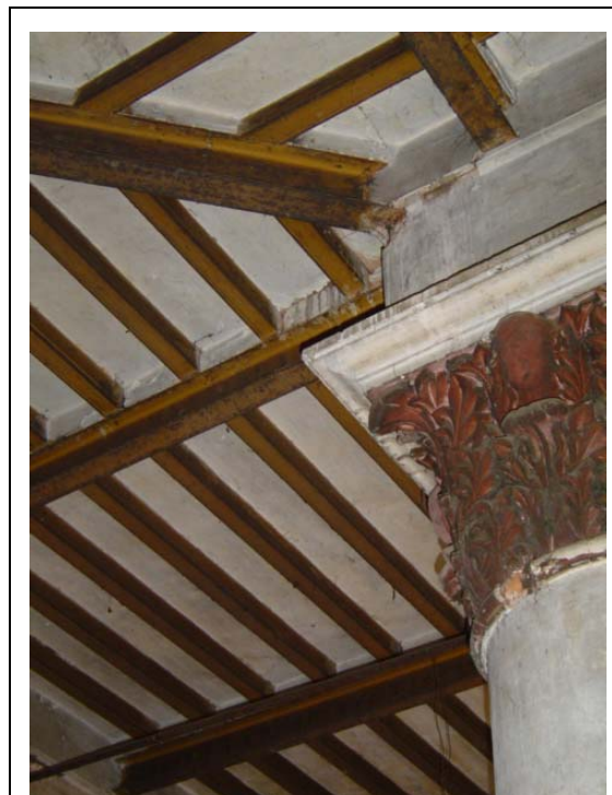
Fig: 19 Ceiling with I beam and decorative column
