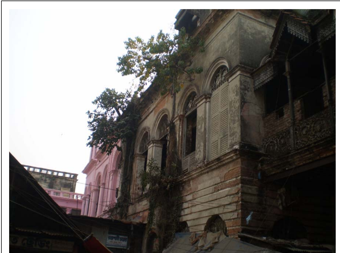
Fig: 17 Central Block (source: Author's collection)
