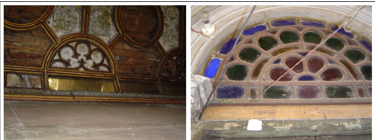
Fig: 22 & 23 Decorative Ceiling work & color Glass (source: student's report)
