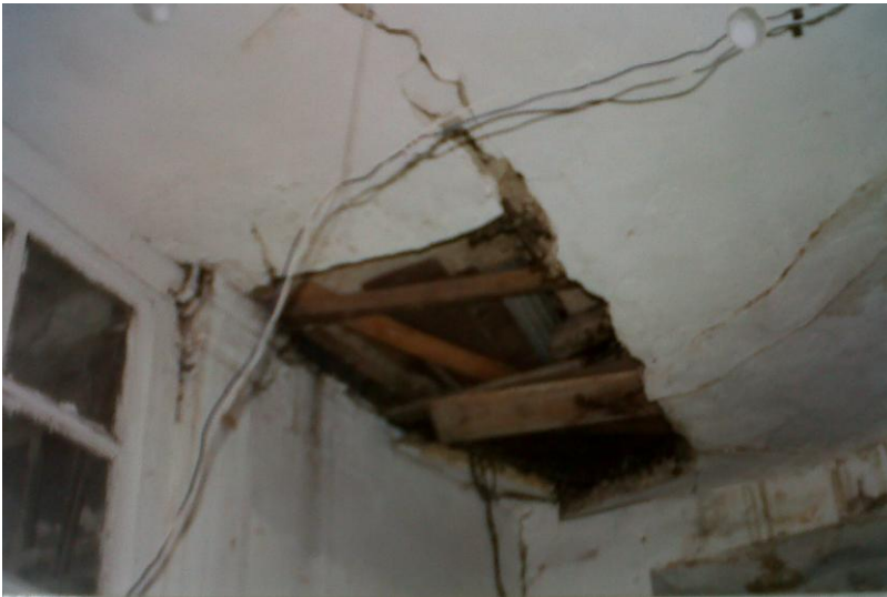
Figure 5: First floor ceiling.
