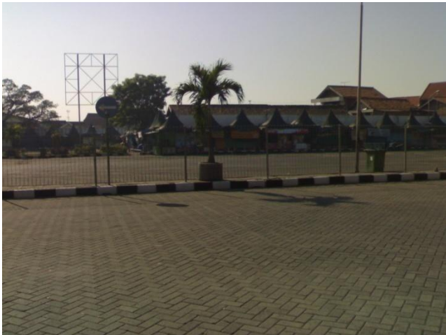
Fig. 74 Bus Parking Area
