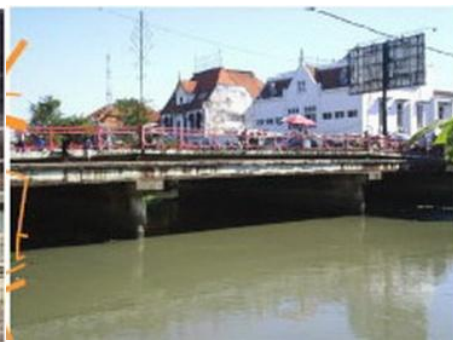
Fig.4 Jembatan Merah (Red Bridge)
