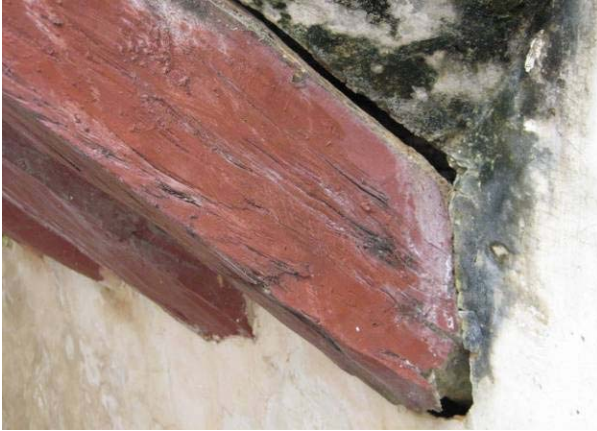
Moisture surfaces under stairs. Rotten wooden ceiling joists.
