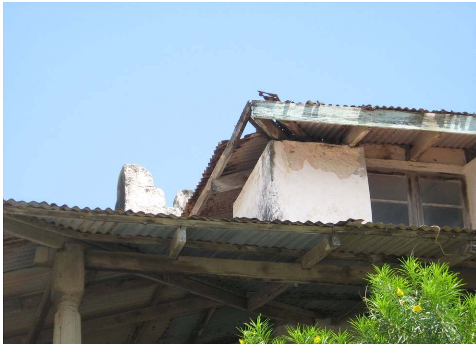
Moisture surfaces under stairs. Rotten wooden ceiling joists.
