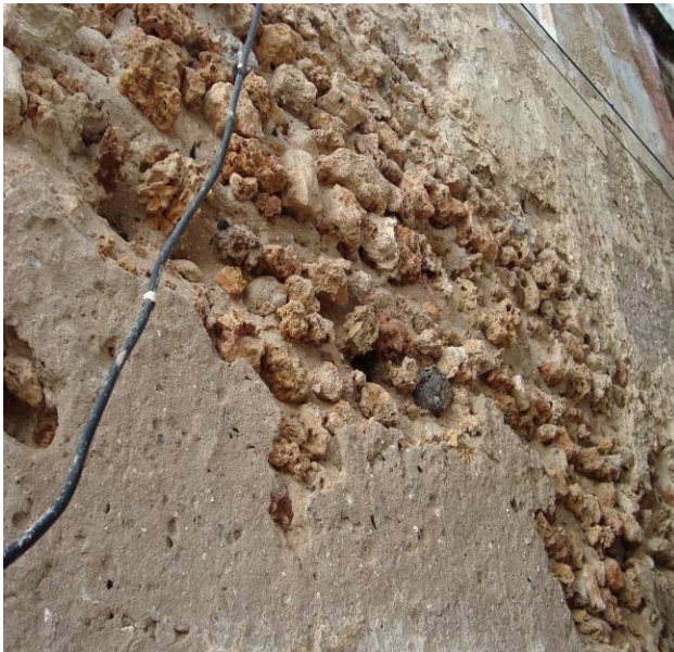
Deteriorated plaster work on the exterior walls
