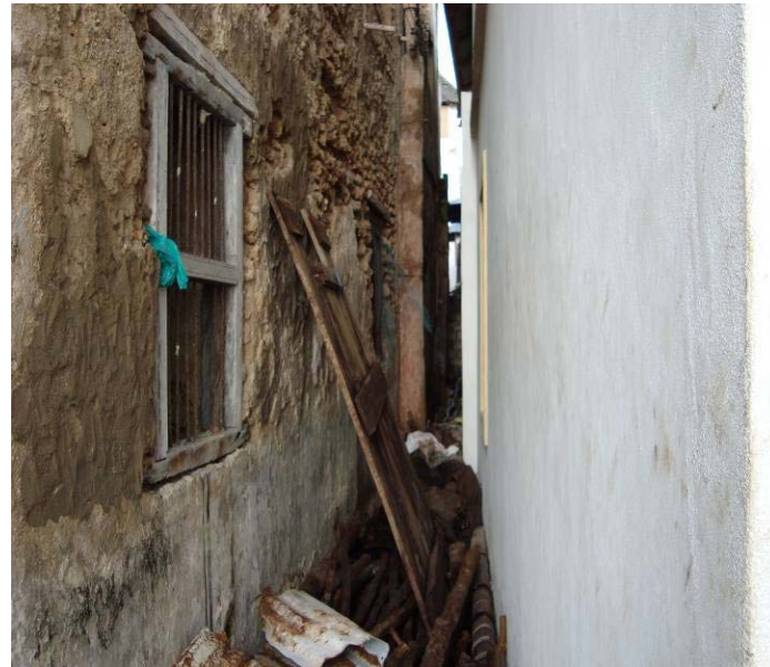
Deteriorated plaster work on the exterior walls
