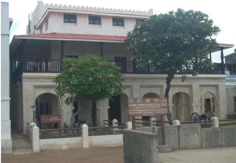
has coral wall approximate 500mm thick bonded in lime Mortar mix.
