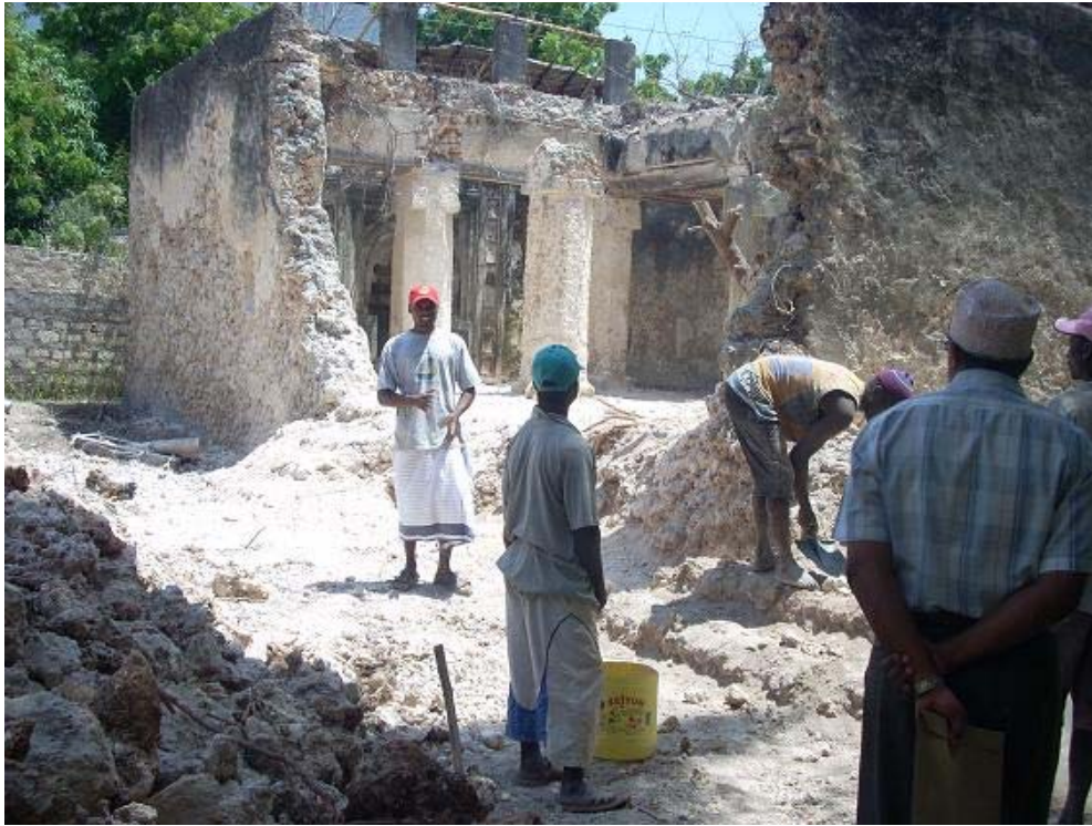
Plate 15. Western façade before reconstruction
