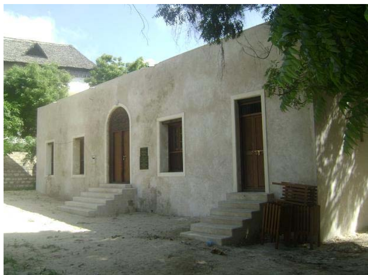
Plate 26.the rehabilitated western facade
