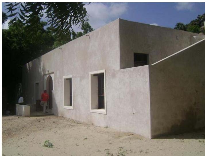
Plate 27.the rehabilitated eastern façade
