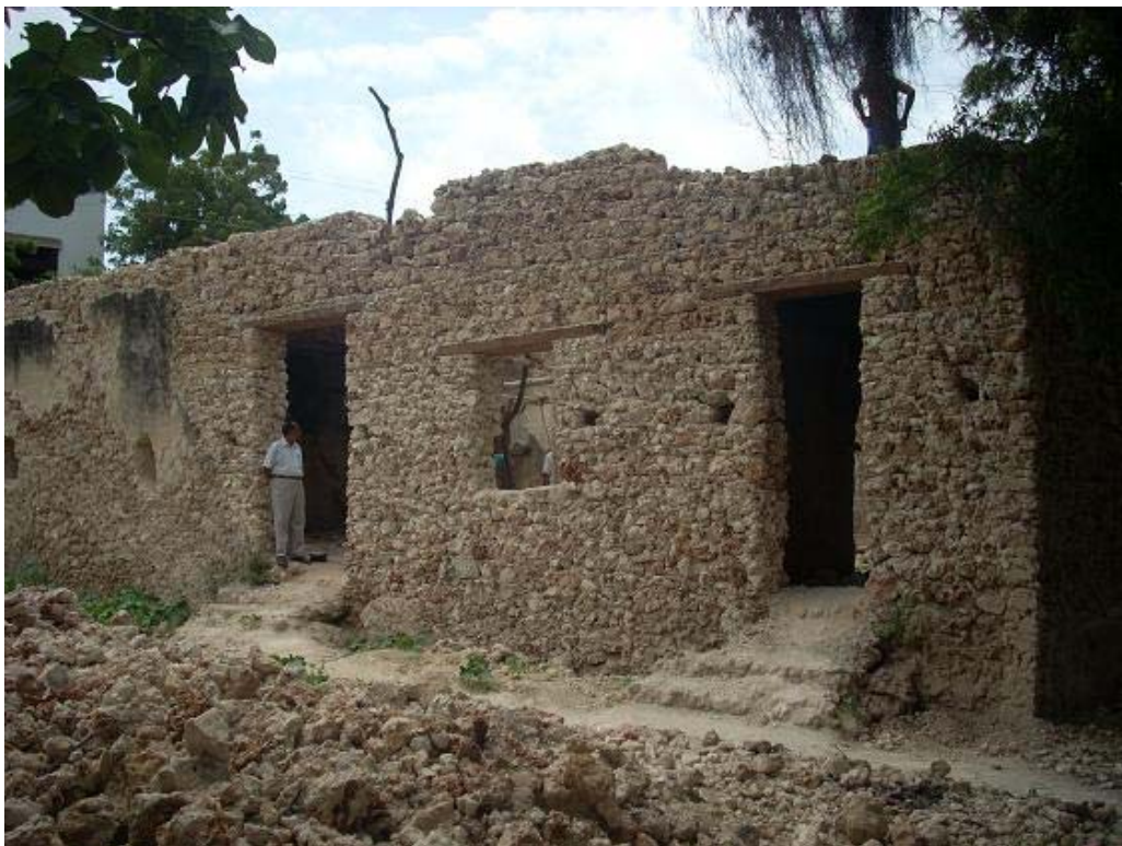
Plate 16. Western façade after reconstruction
