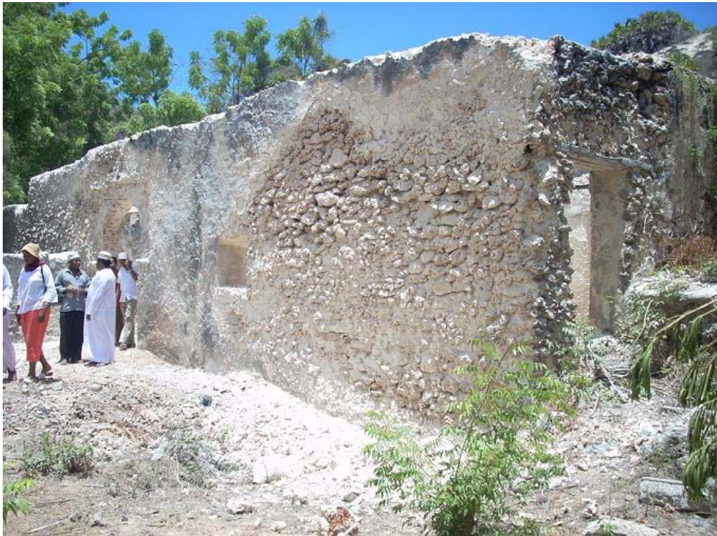
Plate 13. Eastern façade of the mosque as work commenced
