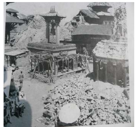
Fig-8, source: book, Patan Durbar Square after 1934 earthquake.
