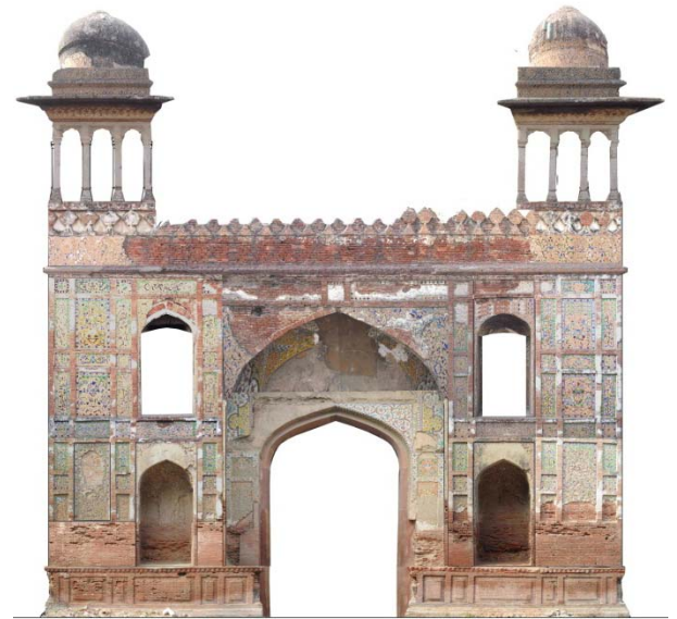
Existing East Elevation of the Gate Way in the Dilapidated Condition
