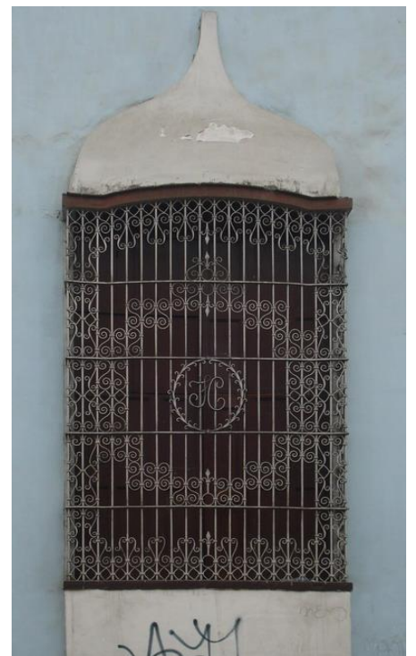
Figure 43: Window of lateral facade
