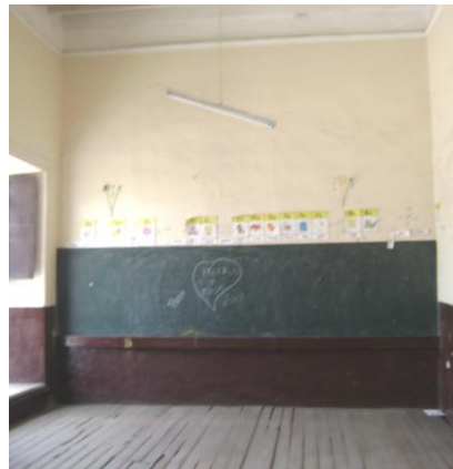
Figure 30: Blackboard embedded in adobe walls
