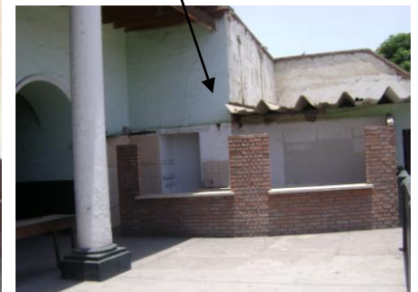
Figure 31: Brick wall needed to be removed
