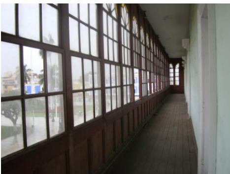
Figure 11: Balcony area – Zone 1
