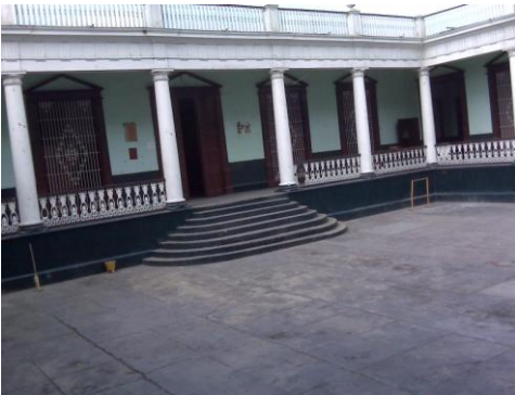
Figure 10: Main yard – Zone 2
