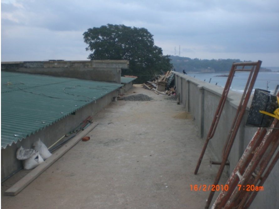
Building being conserved – Modern roof
