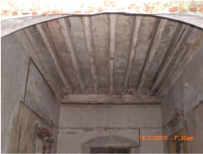
Building being conserved – Roof slab
