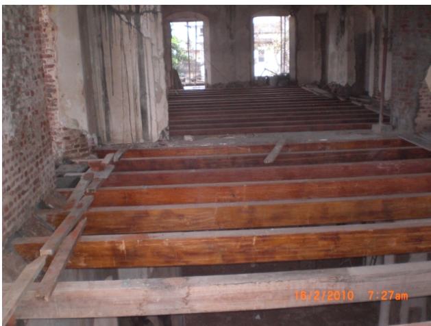
Building being conserved –First floor Timber Deck
