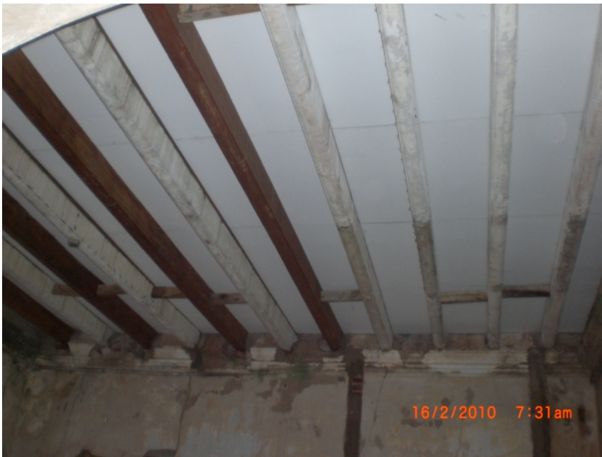
Building being conserved – Slab imitation
