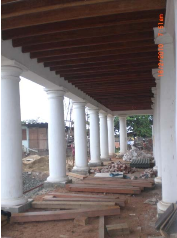
Building Being Conserved –Outer verandah
