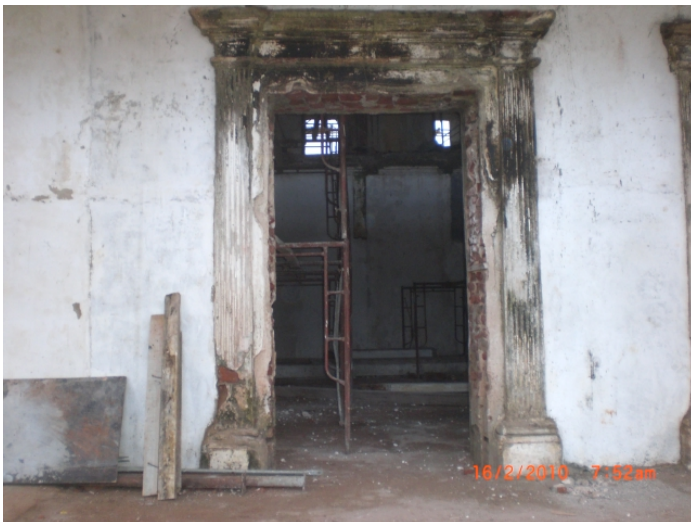
Building Being Conserved –Front Door
