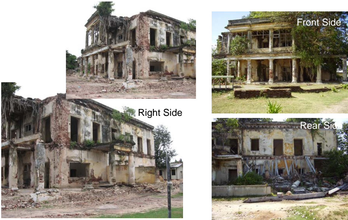
Views of the building in dilapidated condition
