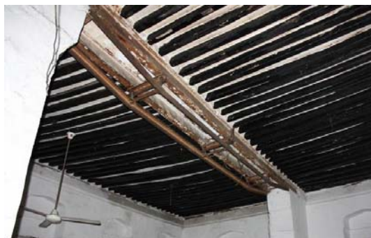
Figure 13 Metal structure to expand span
