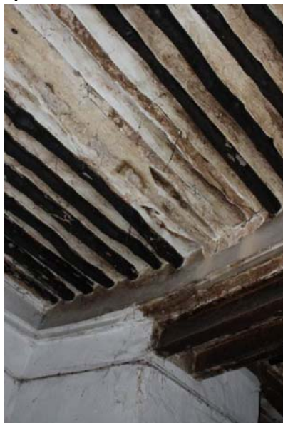
Figure 18 Slab with missing mangrove poles
