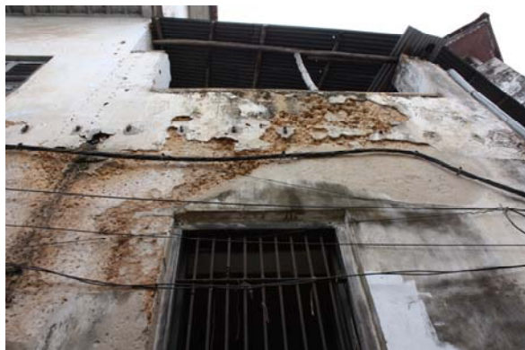
Figure 17 Condition of the wall inside the building
