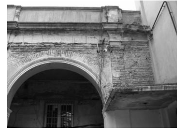
3.view of a lintel system heavy type
