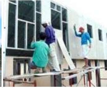
boards are being screwed
