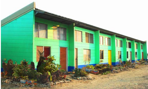
Len Alanzalon & Rosie Mancile's project in Malabon, City. The houses were constructed on a filled-up idle fish pond.
